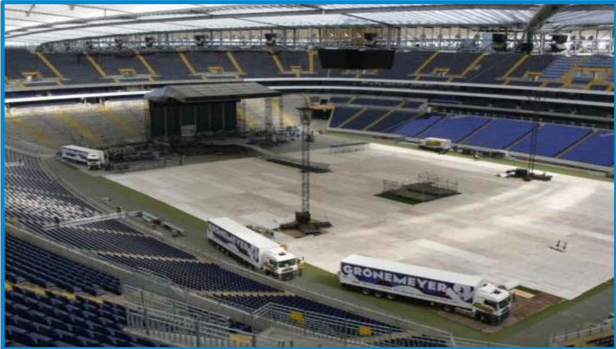
Figure 33 Example truck access pitch Frankfurt Commerzbank Arena, Germany
