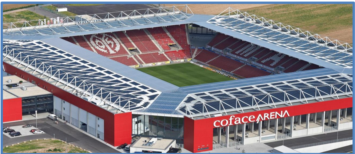
Figure 10 Concrete structure Coface Arena Mainz, Germany
