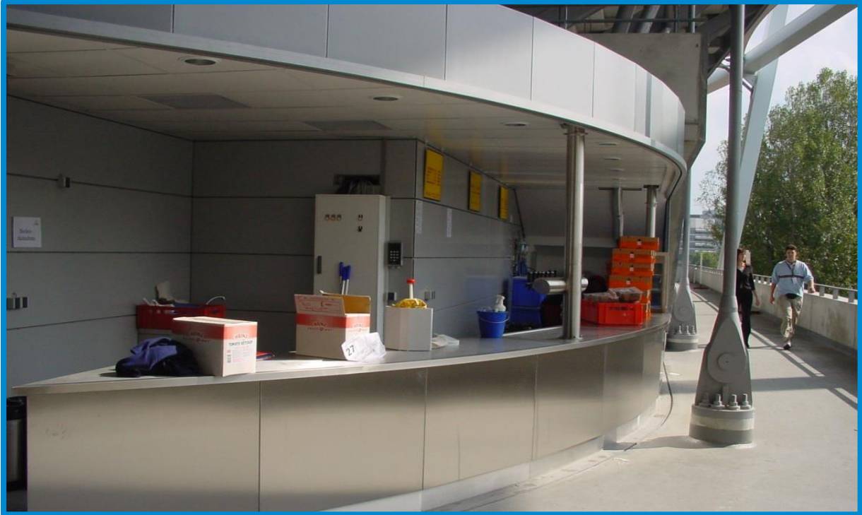
Figure 71 Concession stand Gottlieb-Daimler Stadium Stuttgart, Germany
