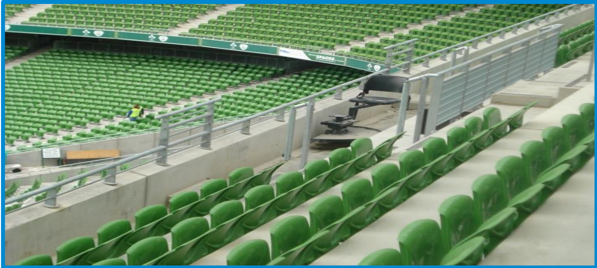
Figure 16 Railings Aviva Stadium Dublin, Ireland
