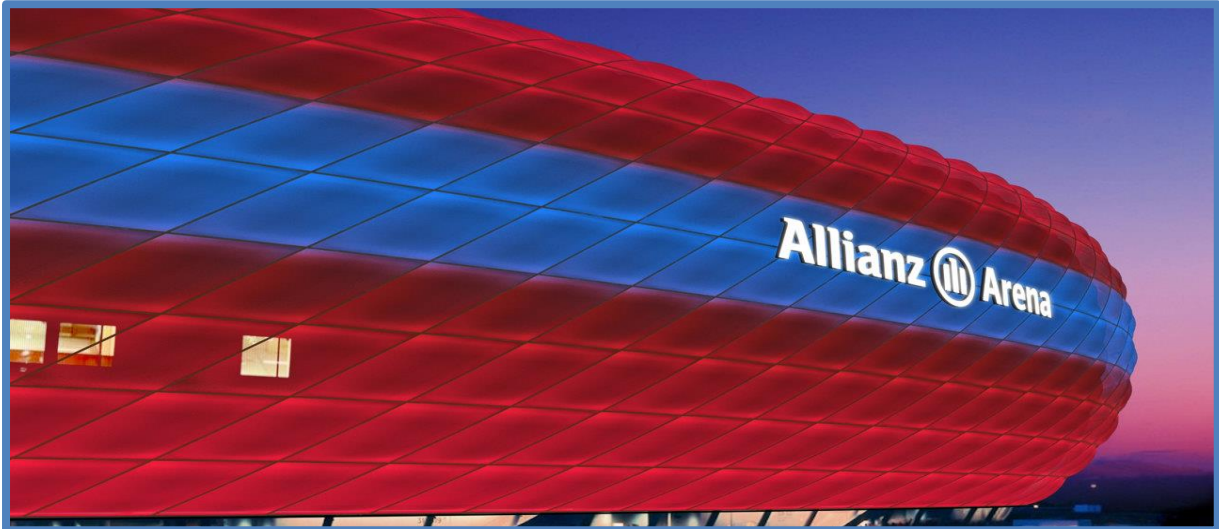
Figure 9 Exterior membrane façade Allianz Arena Munich, Germany
